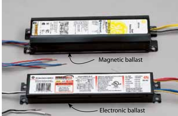
Look at ballast labels for two important ratings: Minimum starting temperature, shown in degrees, and noise rating, where A ranks quietest.
