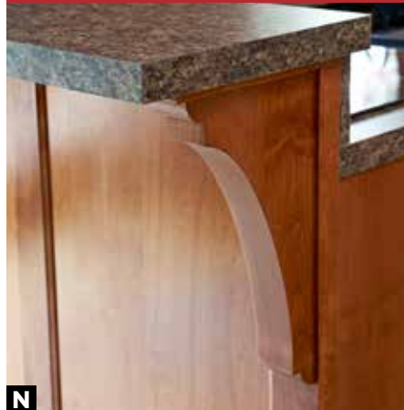
N Shop-made brackets below the snack counter provide a personal touch. You can also buy ready-to-stain brackets in many styles.
