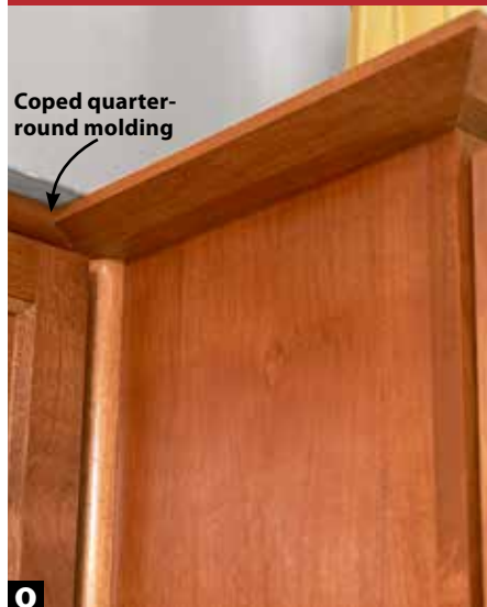
Q Chamfered molding tops the bumped-out cabinets. Flexible quarter-round molding follows the soffit above the cabinets.
