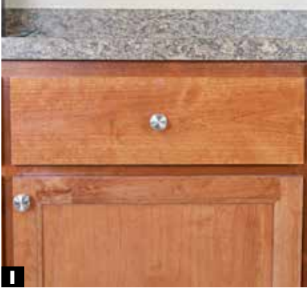
I By installing the cabinet doors first, you can align overlay drawer fronts with doors of the same width.
