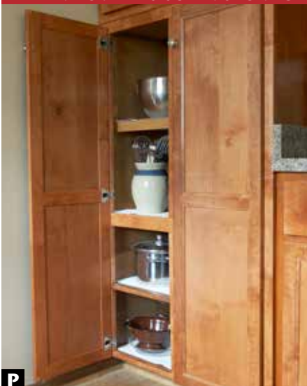
P For the 53"-tall doors on this pantry, we divided the panels with center rails and added a third hinge for support.
