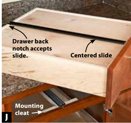
J Centered slide parts automatically center the drawer within the opening. The mounting cleat helps the slide fit this cabinet depth.
