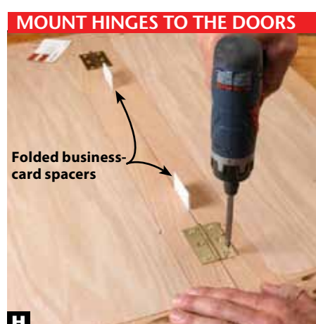
H Center and screw on the hinges between two doors separated by a folded business card that acts as a spacer.
